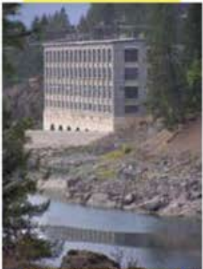
MAIN PPL MONTANA POWERHOUSE
